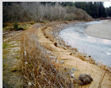
2. Conditions after the first flood. Willows sprouting and taking hold.
